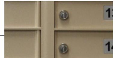
Interlocking, overlapping seams and tight clearances to prevent prying
